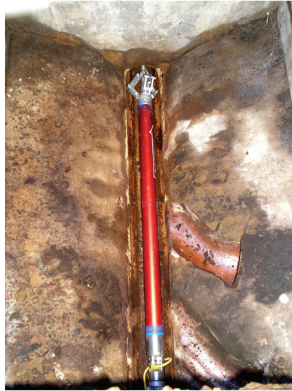
Launching the PipeTrack unit from a manhole.
